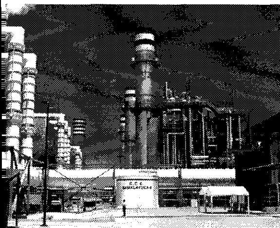
The gas-fired power plant at Samalayuca, Mexico, is another of InterGen's projects. By virtue of its 50% stake in InterGen, the Group has made good on its commitment to enter the power industry.
