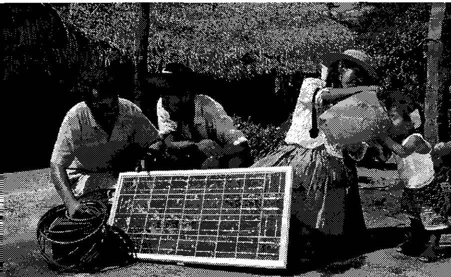
Ernesto Siles points out features on one of the Shell photovoltaic panels incorporated into the 10,000 home solar systems being installed in the rural Santa Cruz area of Bolivia. The systems have been designed for use in remote areas lacking a connection to the national electricity grid.
