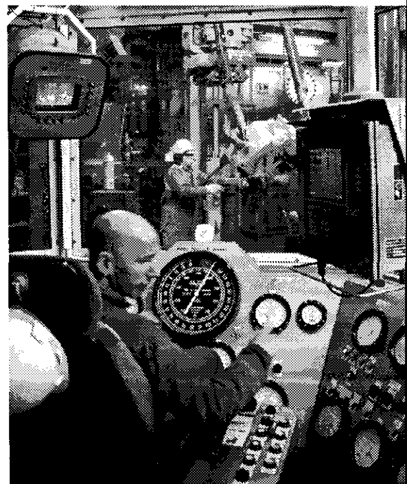
Looking over the driller's shoulder on the Brent Charlie platform, one can see the array of read-outs and dials that enable him to operate machinery safely by remote control. The modern drilling equipment was installed in a major refurbishment that was part of the re-development of the massive Brent field in the North Sea.
